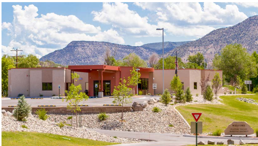
Bighorn Consulting Engineers specified Mitsubishi Electric VRF zoning systems for the Plateau Valley Medical Center.
