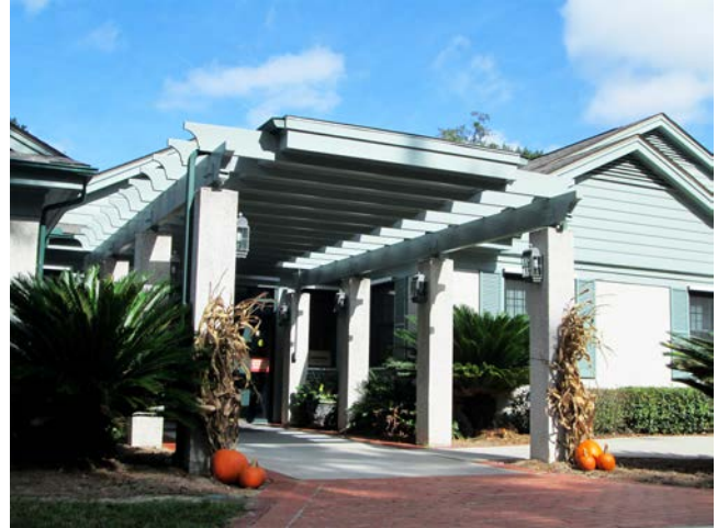
One engineer's decade-long interest in VRF zoning technology began with an HVAC installation in Hospice Savannah.
