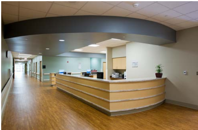
HVAC systems in hospitals face specific challenges.
