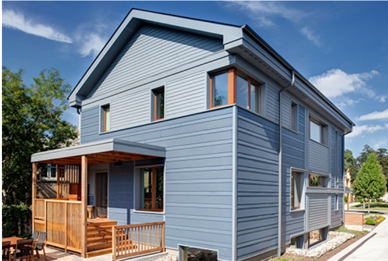
Tom Bassett-Dilley Architect, Ltd., designed this ultra-efficient Passive House in River Forest, Ill., using two Mitsubishi Electric Cooling & Heating mini-splits for heating, cooling and dehumidification.
