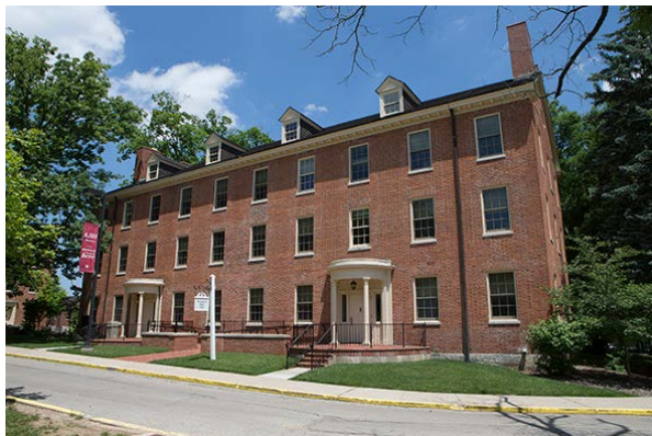
The exterior of the Elliot Hall dormitory at the Miami University of Ohio.
